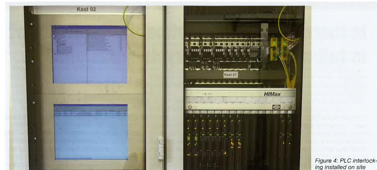
Figure 4: PLC interlocking installed on site
